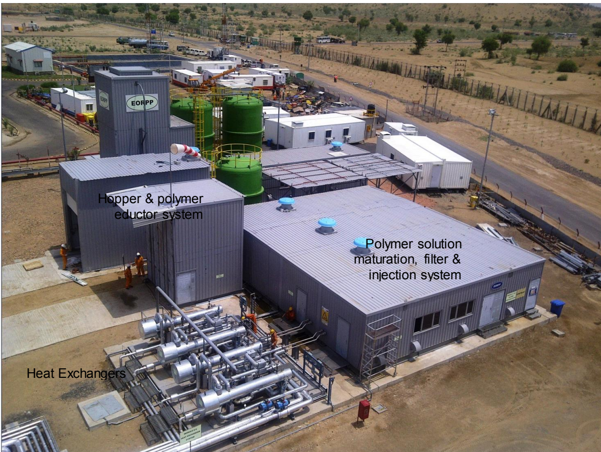
EOR Pilot Facility
